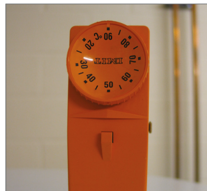
EnergyPro SHWL Plus: turn the pipe thermostat to achieve 50 °C return at the cylinder
