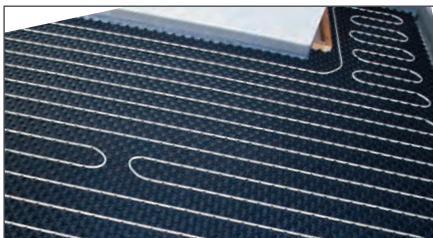
LoPro™ Max – castellated panel and self-levelling compound covers the entire floor
